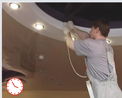
Installation of the ghost tape
