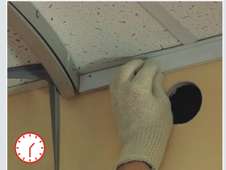
Mounting of the construction, installation of the plastic profiles on the other walls
