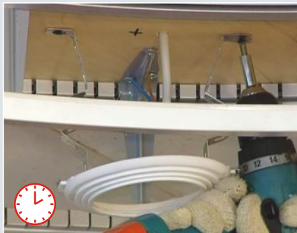
Installation of the universal platforms
